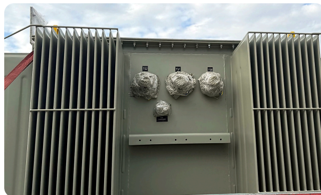
Cable-connection side with protected terminals
